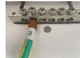
▲ Figure 4.10 Grounding Terminal on Heat-Sink
