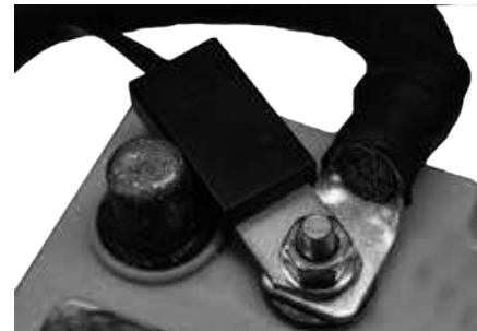
Fig 2.5(b) Temperature Sensor Installation
