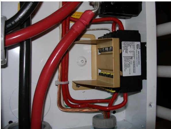
Din Rail mounted breakers
